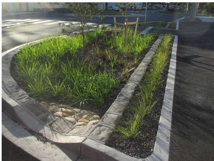
Figure 6 : Stormwater biofilter (Payne, 2017)
