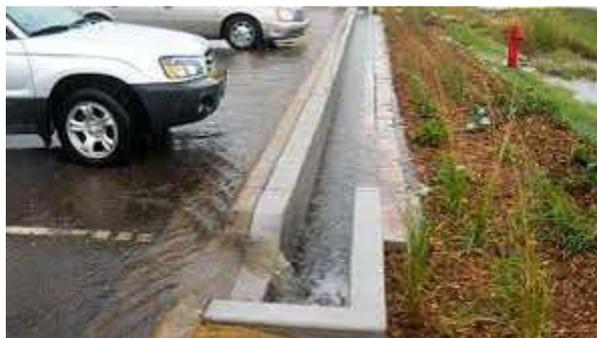
Figure 8 : Exemple d'un level spreader device (Minnesota Pollution Control Agency, 2014)
