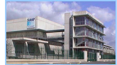
Station Seine Centre (SIAAP)
